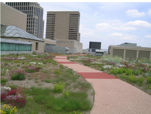
The green roof atop the Lazarus Government Center in downtown Columbus, OH keeps the building cooler and recycles rain water for toilets.
